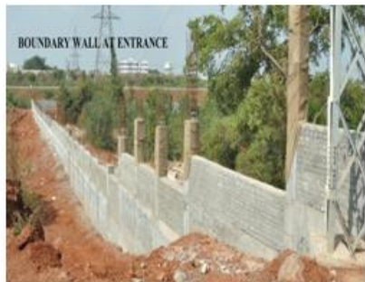
BOUNDARY WALL AT ENTRANCE
