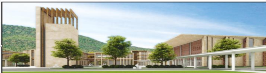
LIBRARY & ADMIN. BLOCK & AUDITORIUM – AIIMS MANGALGIRI, A.P.
